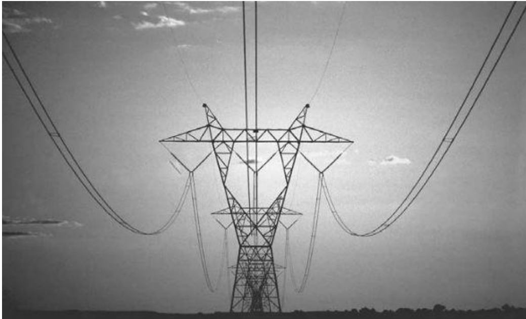
Figure 40: High-voltage transmission lines [51]
